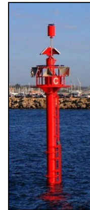
Figure 3-8c Spar Buoy
